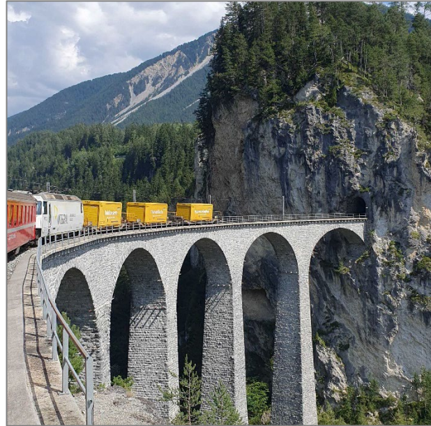
Landwasser viaduct railway bridge
