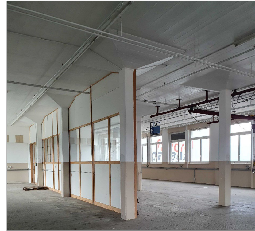
Favarol Papaux factory, Treyvaux Reinforced concrete structure
