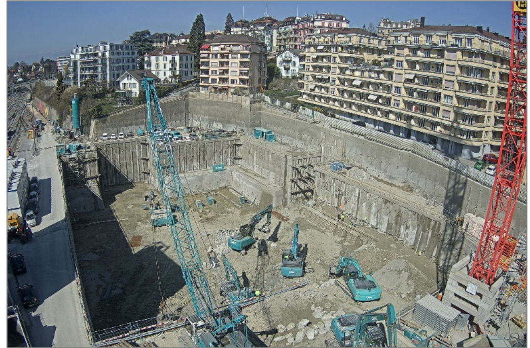
Elysée/mudac, Plateforme 10, Lausanne excavation supports
