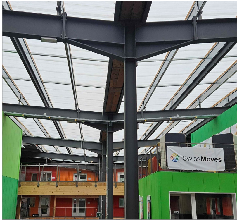
Halle Bleue, Blue Factory, Fribourg steel frame
